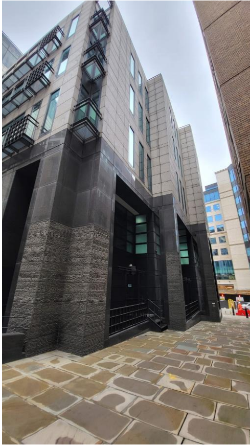
Image 6: The southern elevation of the southern block within Ashentree Court.
