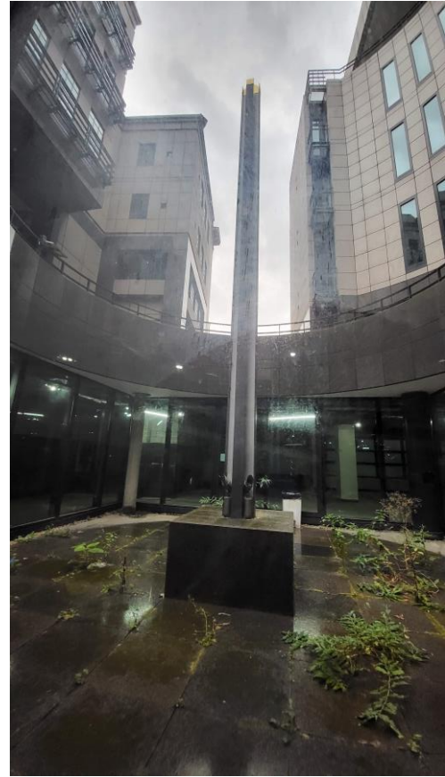
Image 7: The base of the existing lightwell in the centre of the courtyard
